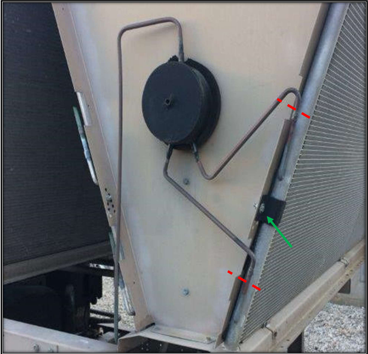
Figure 3. Back of Chiller: Cut existing receiver lines as shown in Red. Unbolt the coil at 4X locations as shown in Green.
