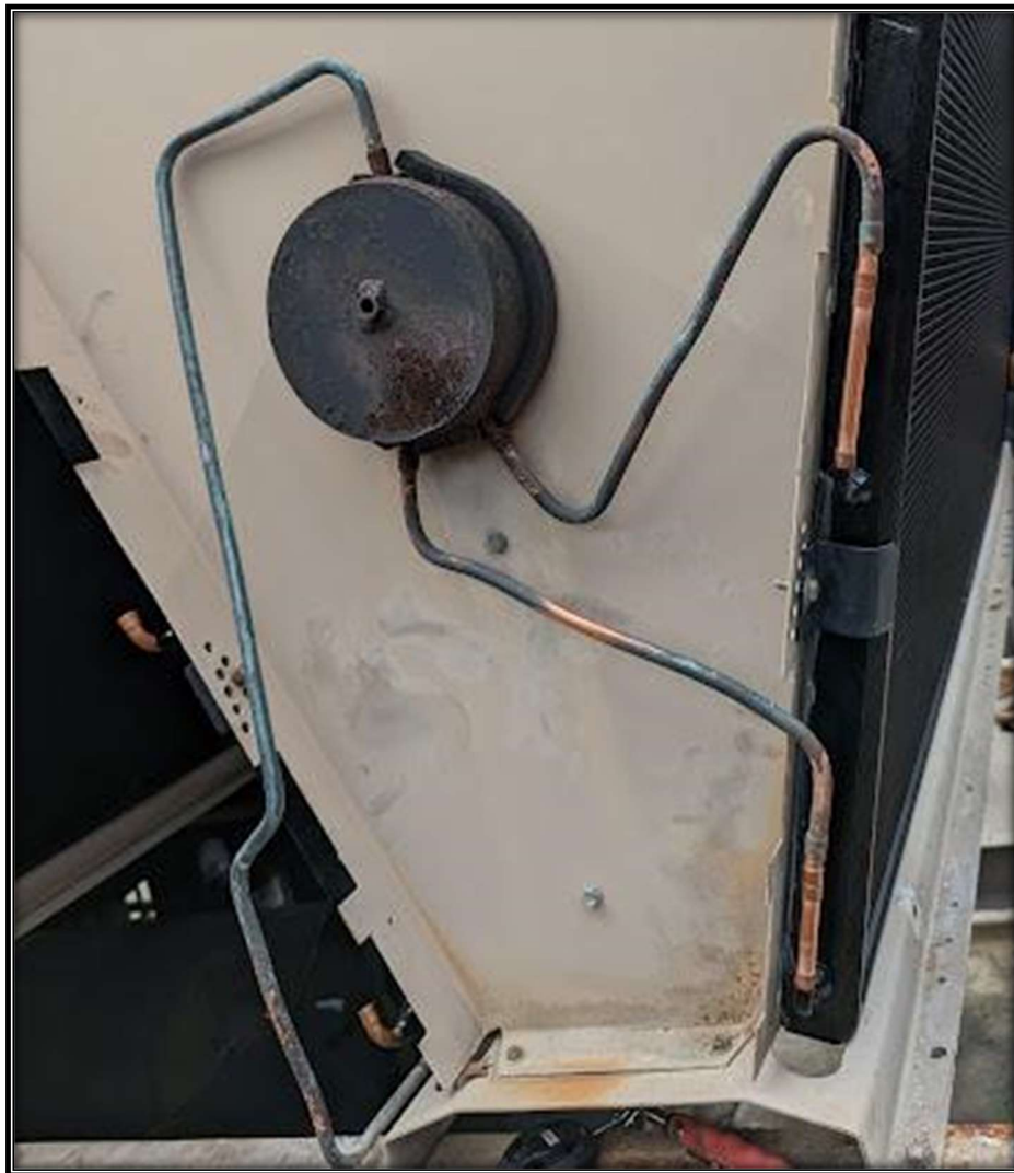
Figure 5. Back of Chiller: Solder receiver lines as shown.
