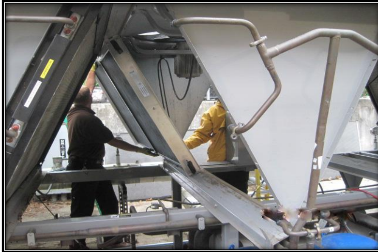
Figure 6. Coil Installation
